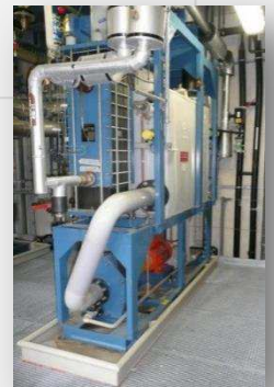
Pump skid with condenser
